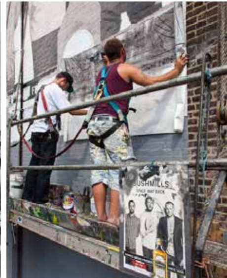
Our painters pouncing a sign space in 2012
