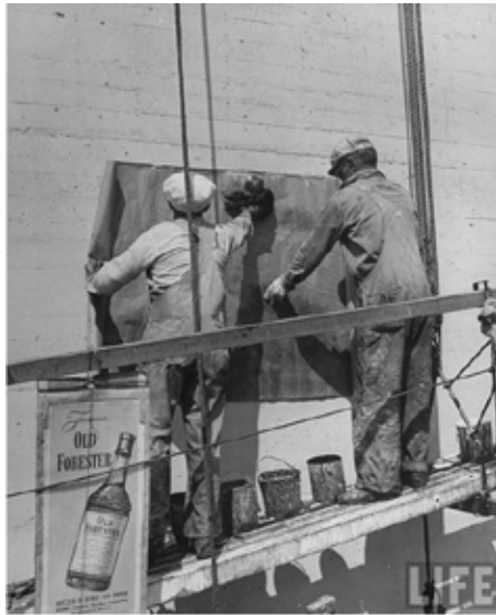
"Pouncing," a process of prepping a sign space 1930's
